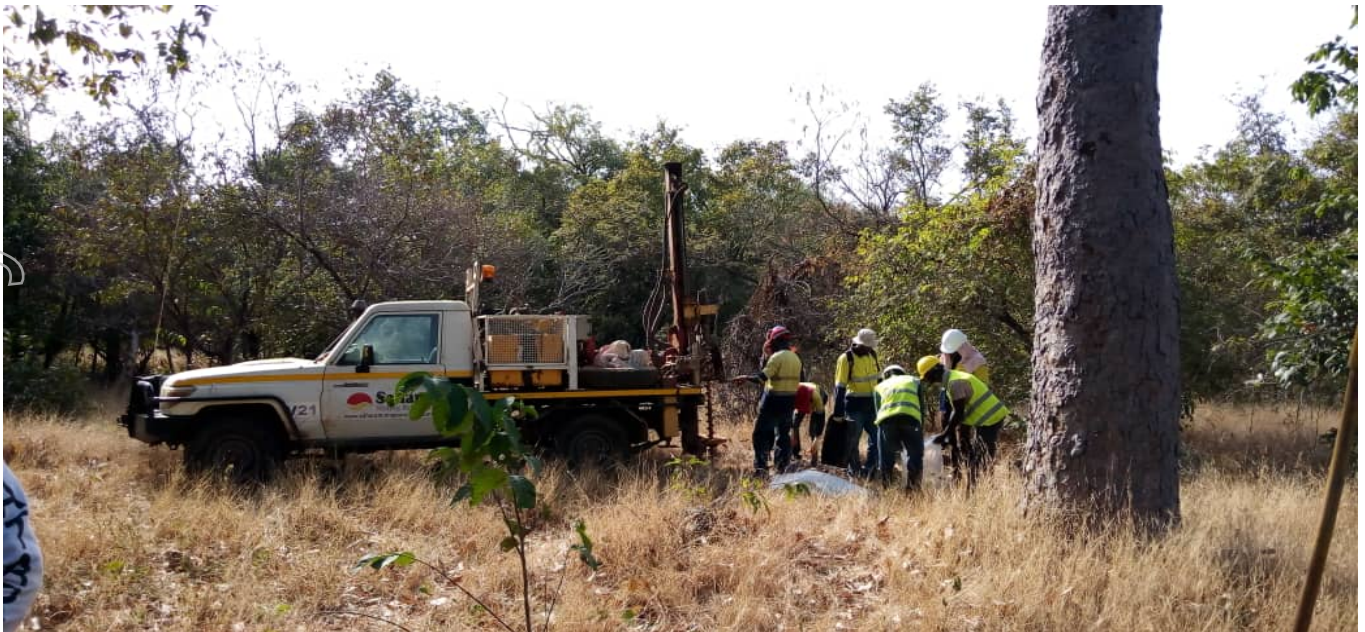
Figure 5: Drill Rig & Crew undertaking Drilling Operations
