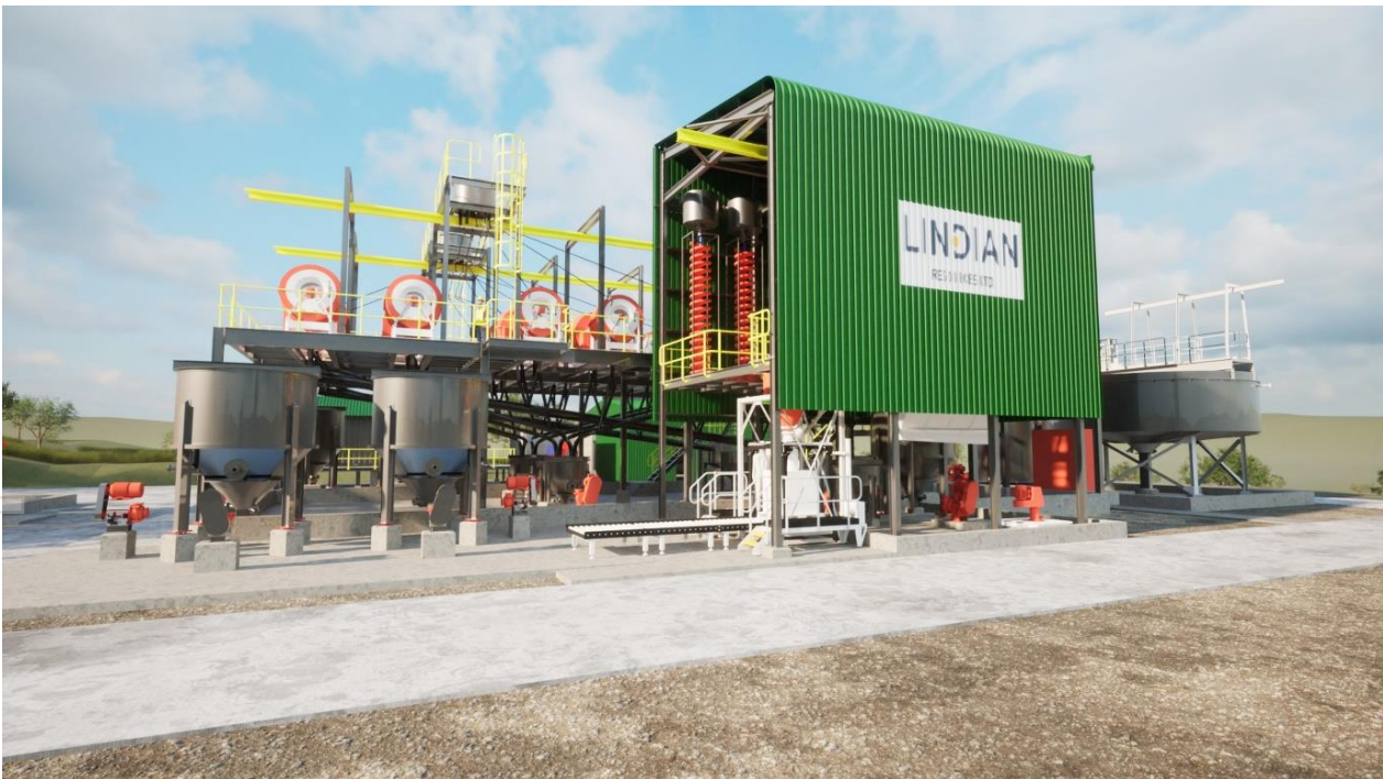
Image 6: Side view of the recovery circuit and concentrate filter press and packing shed and tails thickener.
